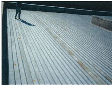
Atiamuri Roof—Mighty River Power
