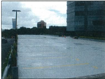
Car Parking Deck
