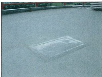
Dairy Powder Tower Roof
