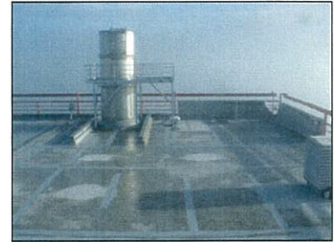
Dairy Powder Tower Roof
